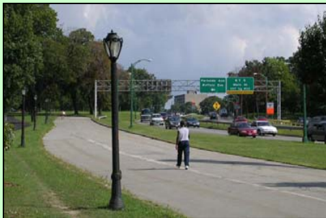
Figure ii – The Scajaquada Expressway now cuts through Delaware Park
